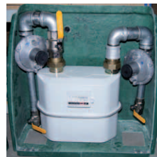
Typical U25 Low Pressure Metering System with OPSO and UPSO
