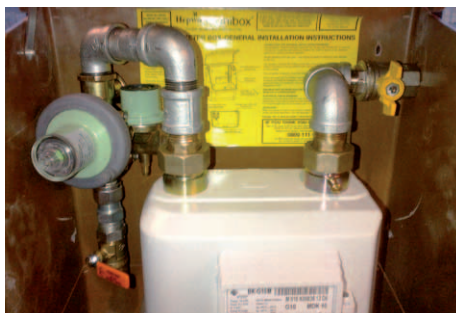
Medium Pressure U16 Meter Module in a Unibox
